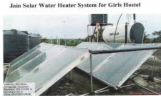
Jain Solar Water Heater System, close Loop 1000 LPD
