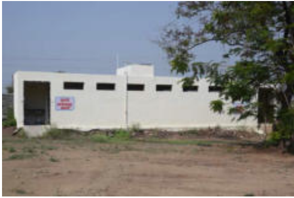
Boys Toilet Block
